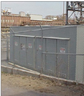
Metal Enclosed Shunt or Filter Bank
